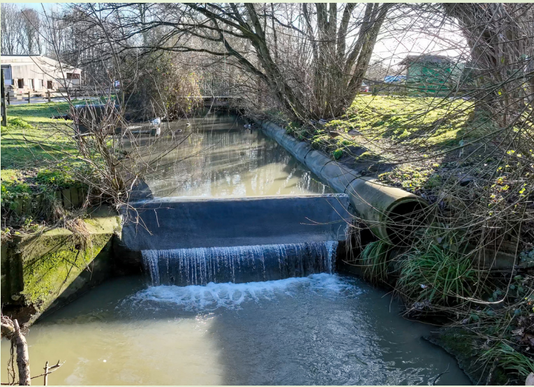
Figure 3. Drone footage of the weir at Standalone Farm
