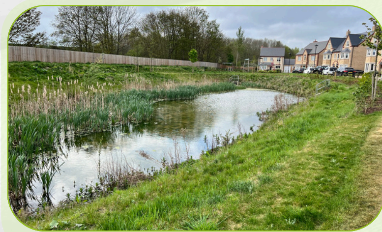
Figure 3. Fairfield Attenuation Pond
