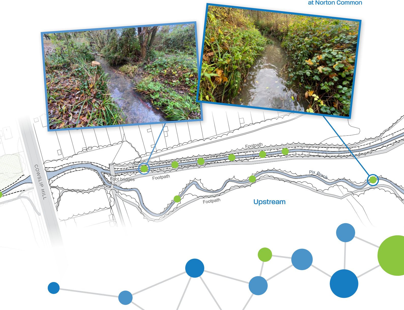
Examples of existing channel at Norton Common
